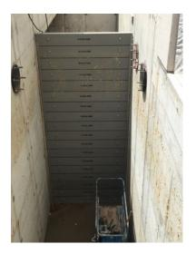
When needed, guide frames include a specially designed neoprene seal with a dual-edge profile. This creates targeted contact pressure against the stop log for a strong, reliable seal. Most stop logs include a full-length neoprene seal along the sides.
